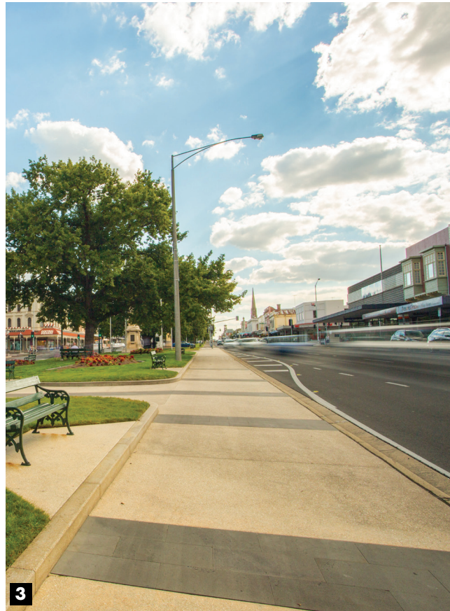
3 5 7 Sturt Street 9 10 Various buildings
